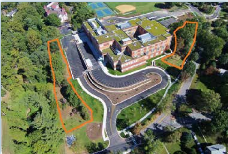
On-site forest conservation areas at Silver Creek Middle School.
