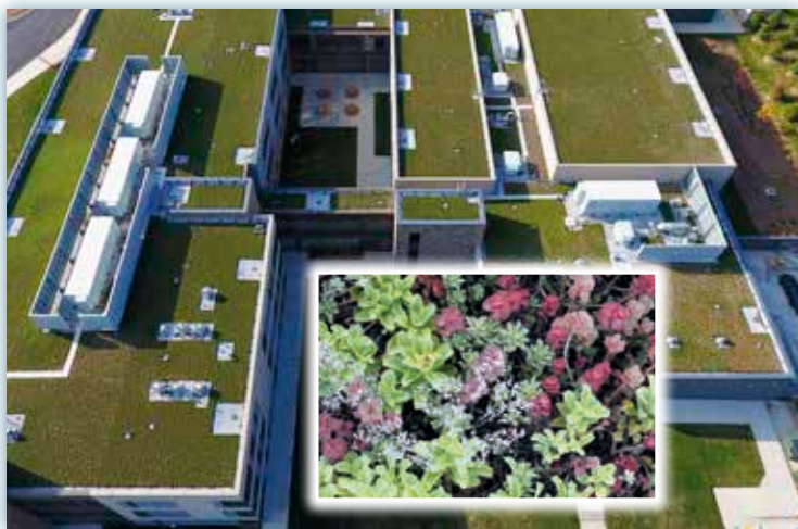
Green roof at William H. Farquhar Middle School. [Hord Coplan Macht, architect; photography by Patrick Ross] Inset photo shows types of vegetation used on green roofs.
