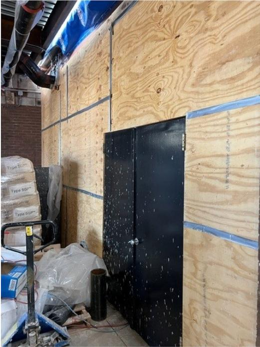
Photo 9: Door to Containment (Construction Side)
